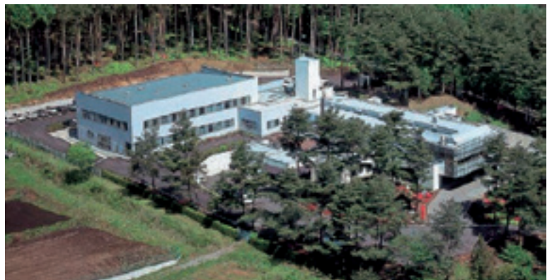
Product Development Center (Minowa-machi, Kamiina-gun, Nagano Prefecture)
