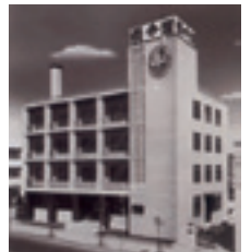
Former Head Office Building
