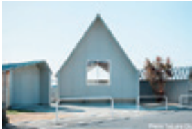
e-Collaboration Tsurugashima (Tsurugashima-shi, Saitama Prefecture)
